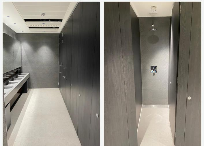
Unity Full Height SGL shower cubicles were specified for the changing rooms. The full height floor to ceiling cubicles are ideal for creating complete privacy. The doors and panels are manufactured using Solid Grade Laminate (SGL), ensuring the shower cubicles are completely water resistant and hardwearing.
